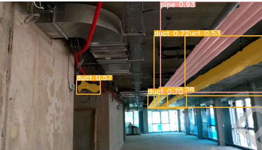
Figure 11: Failure case: Low lighting conditions (under 300 lux) and low contrast ( \sigma = 15 ) prevents reliable edge detection.
